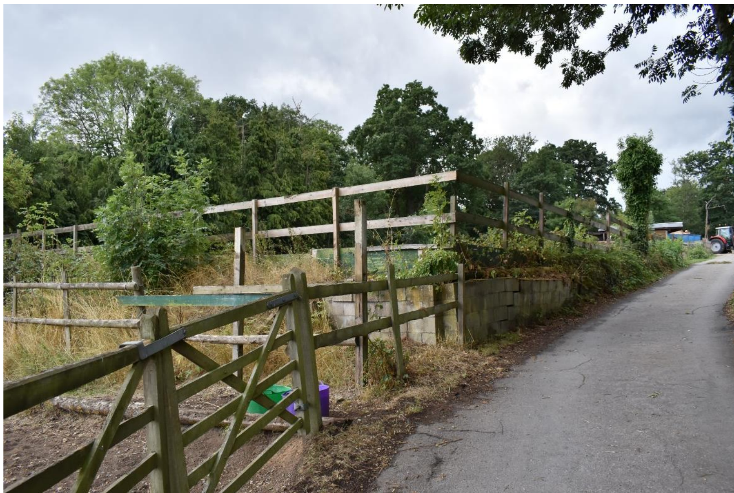
Plate14: View of the retaining wall of the dressage school (facing S).
