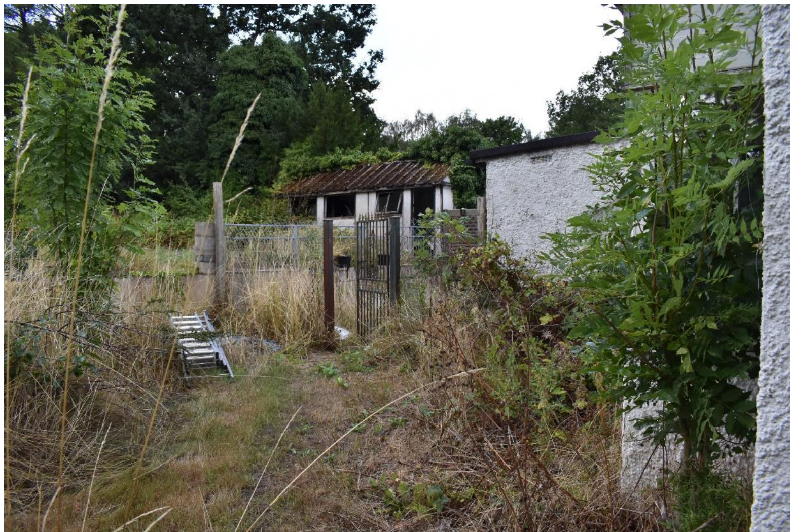
Plate 18: View of retaining wall at the rear of the house (Facing W).
